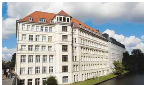
Office property Sonnenallee
